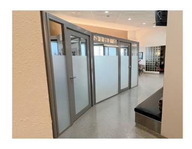
field-fit and can accommodate variations in floor and wall measurement. Also, by using a single installation team, the project was finished in one week as opposed to dragging out for weeks if traditional construction methods had been used.
